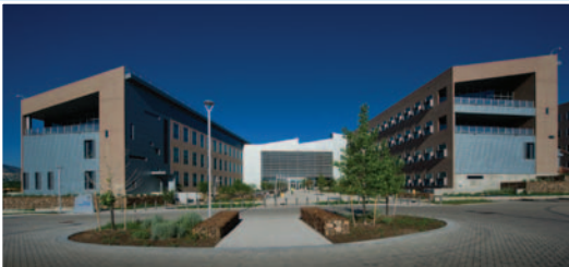
The Research Support Facility at NREL is a living model for smart energy use.
